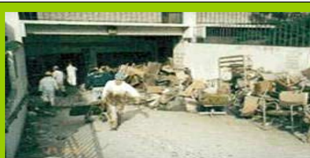
Figure 1: Remediation of an office building
